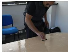
7. Slightly moisten the backing and apply light pressure with the squeegee provided (over the entire surface, starting from the centre and working towards the edges).
