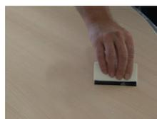
8. Apply more pressure with the squeegee to drive out the water completely (over the entire surface, from the centre to the edges). To guarantee optimal adhesion, the water must have totally disappeared.
