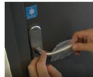
3. Apply the film (uncut area) to the convex part of the handle (part rounded outwards). Apply pressure with your thumbs.
