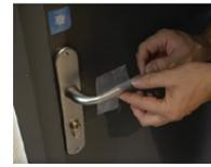
4. Apply the pre-cut strips one by one around the handle. Apply pressure with your thumbs. First apply the strips underneath, then the strips on top.
