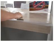
3. Apply the film using the squeegee provided, making a 45° angle between the surface of the squeegee and the film.
