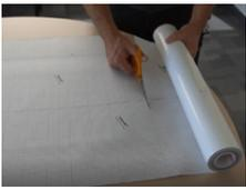
1. If the surface is square or rectangular, cut directly to the right format (690x690mm for a 700x700mm table). Make 5mm rays in the corners. If the surface is complex in shape, and only in this case, leave an surplus which will be cut and removed at the end of the installation.
