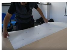
3. Apply the film with its liner on the wet surface (liner upwards).
