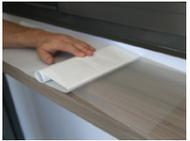
2. Remove about 2 cm of the liner and apply the film. Then remove approx. 20 cm of the liner (without sticking the film).
