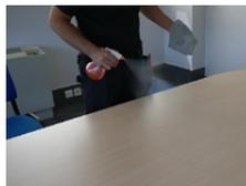
2. Moisten the substrate with plenty of soapy water (washing-up liquid approx. 5-10%) using a spray or atomizer.
