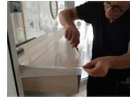
5. Cut off the excess or rewrap the field to the underside of the table. If cutting backwards, cut with a cutter (3mm back from the edge of the support - do not press too hard, otherwise you may scratch it). If overlapping, leave at least 3cm on the underside of the table.
