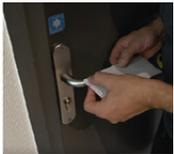
1. Measure the length of the handle to be protected and cut off the excess film. If the circumference of the handle requires it, also re-cut the strips to prevent them from overlapping too much.
